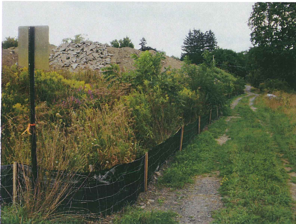
Photograph of filled in channel along west property boundary. August 24, 2011.
