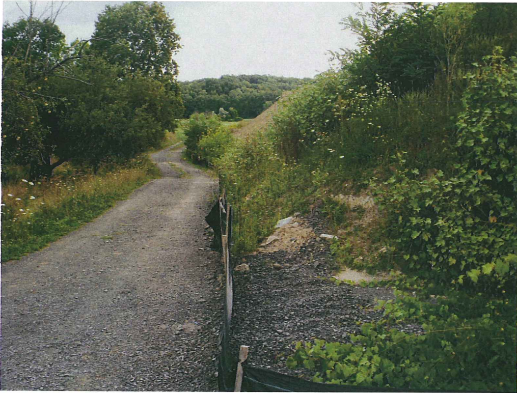
Photograph of the southwest corner hillside and silt fence. August 24, 2011.
