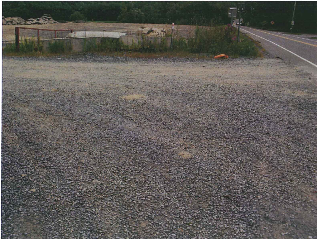
Photograph of stabilized construction entrance. August 24, 2011.
